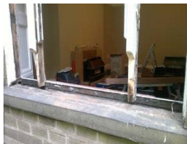
Frame and cill routed to expose sound timber
