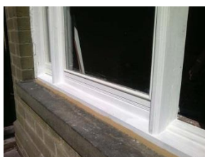
A traditional repair in situ
