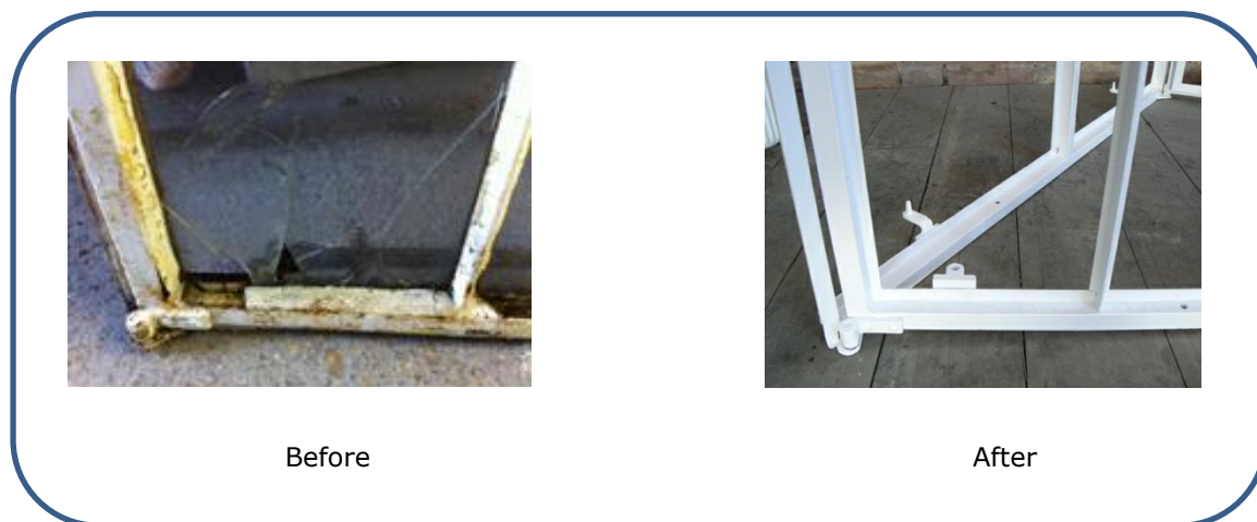
Fig 6 Example of metal repair
