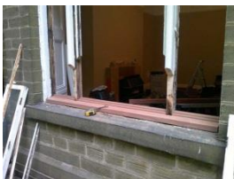
New timber spliced into the frame and made good ready for decoration
