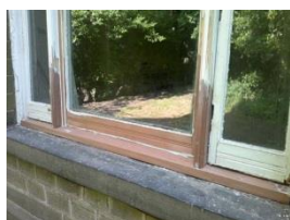
New timber spliced into the frame and made good ready for decoration
