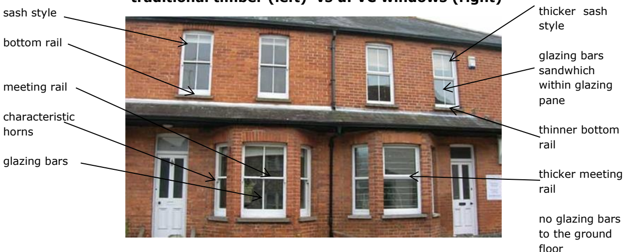
Fig 8: Example of traditional timber (left) vs uPVC windows (right)
